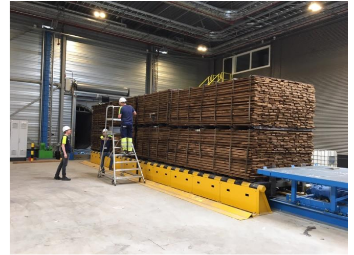
Arnhem plant interior – Reactor 3 loading
