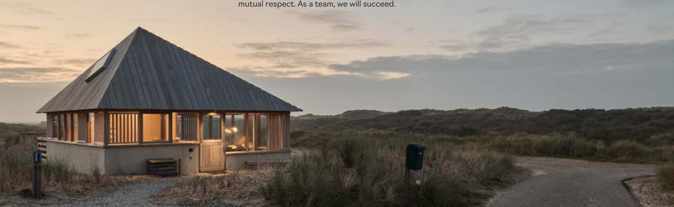
HOUSE IN THE DUNES / TERSCHELLING, THE NETHERLANDS / MWA HART NIBBRIG / KOLTHOF BV
