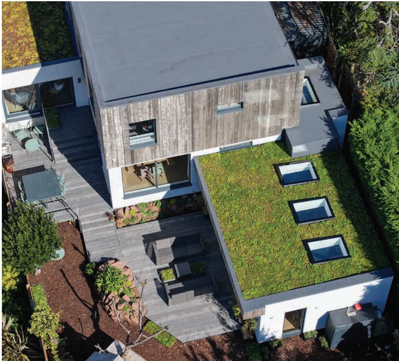
Residential House, Wirral, UK. Supplier: James Lathams. Architect: Bromilow
